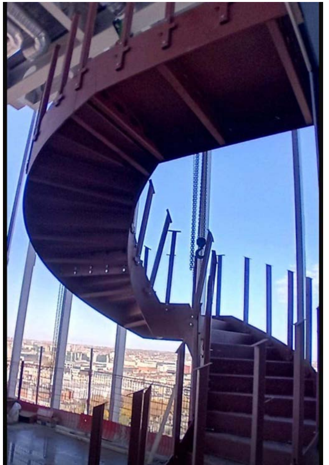
Full site installation by our qualified steel erectors.
