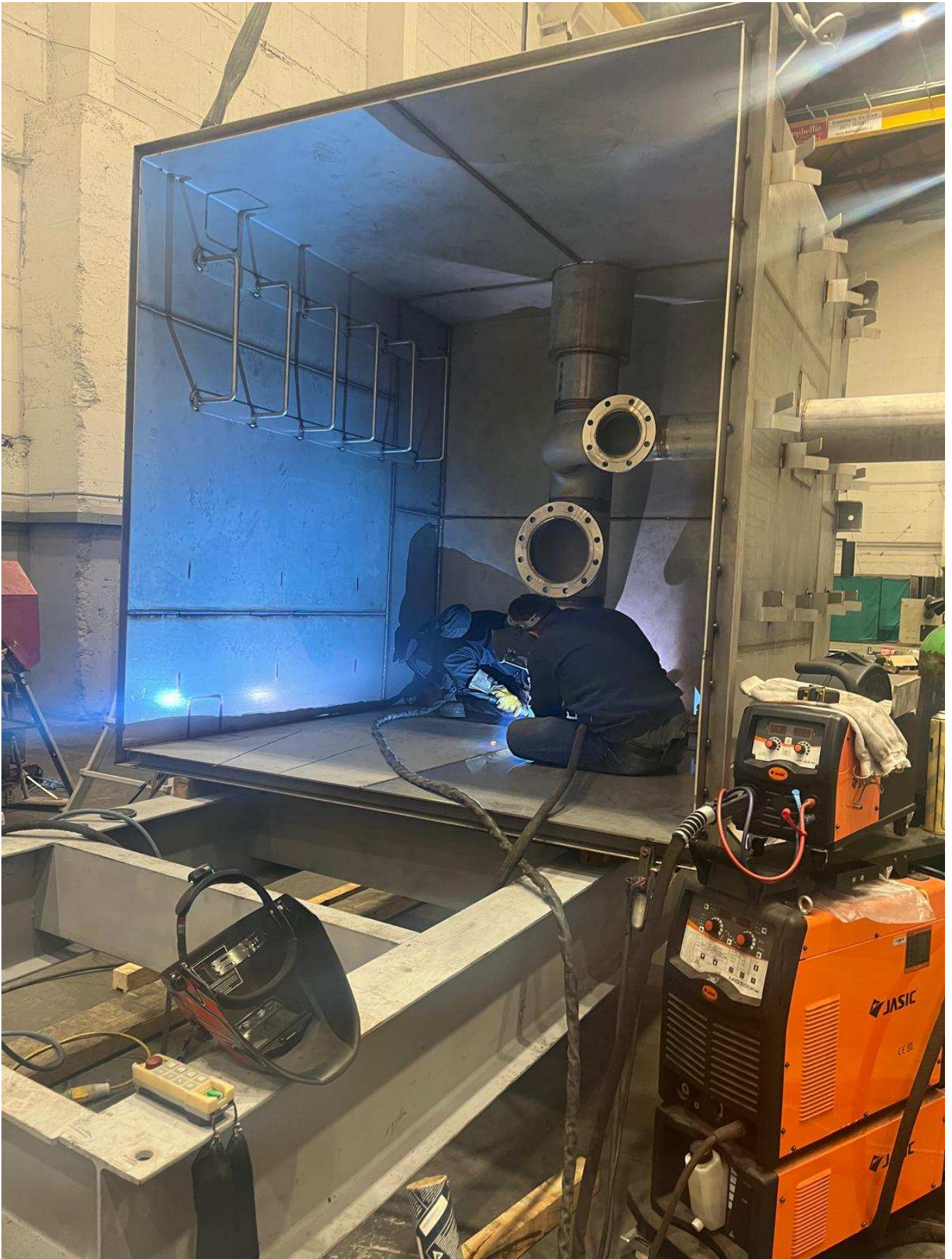
Large stainless steel Inspection chamber being manufactured for Astellas Tralee.
