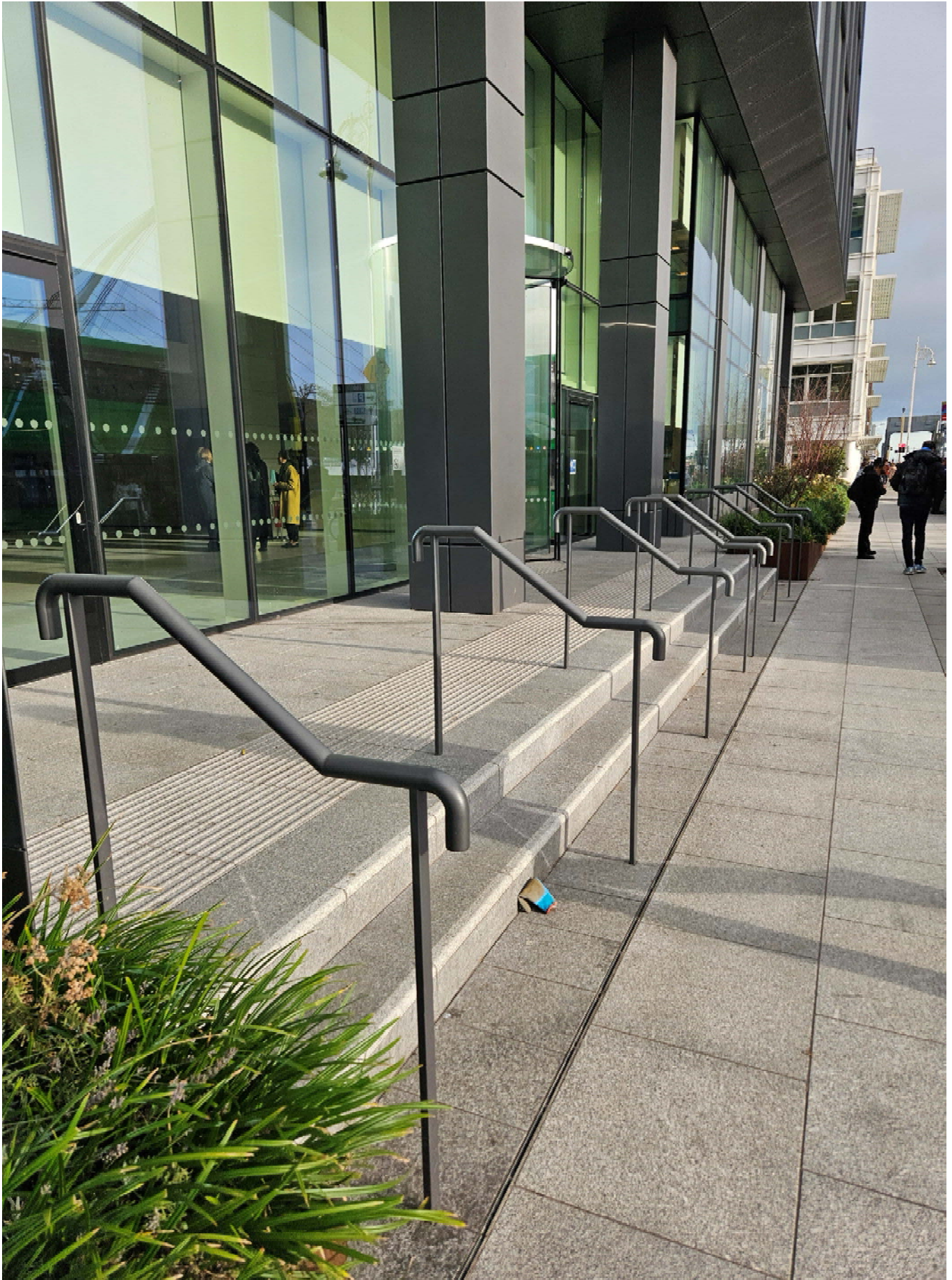
Galvanised and powdercoated entrance rails fitted to North wall quay.
