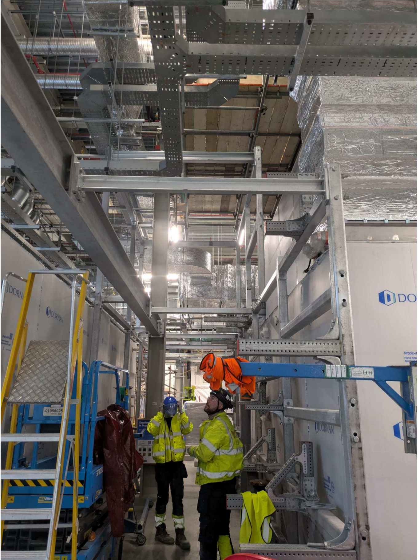
Modular Pipe Racks , design , fabrication, galvanising, delivery and installation.
