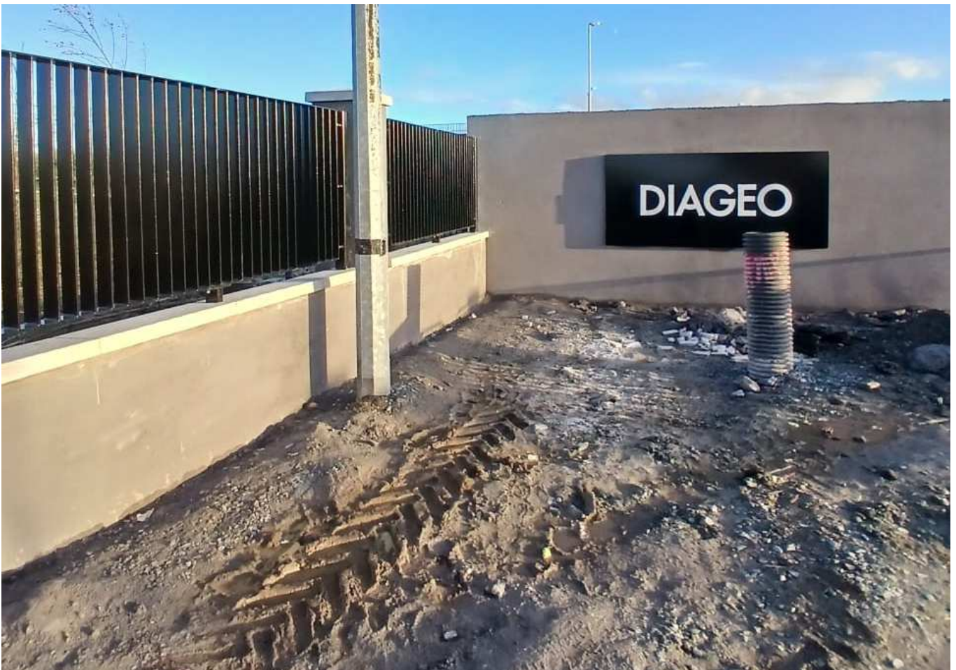
Access stairs, balustrade and stainless steel handrails to the security office and perimeter railings to Diageo processing plant in Kildare.
