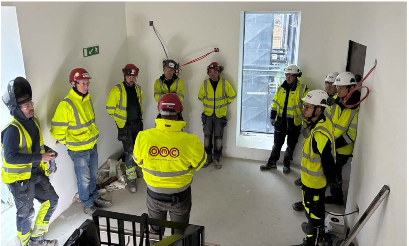
Site supervisor Ruairi Kelly pictured here with his crew in AstraZeneca Pharmaceutical. The crew are receiving a debriefing and toolbox talk from Martin O' Boyle & Laura Gleeson following a quarterly directors walk in AstraZeneca.
