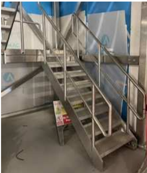
Astrazeneca Dublin. OMC installed stainless steel access platforms, Access stairs, Access ladders, lifting beams and galvanised access platforms.
