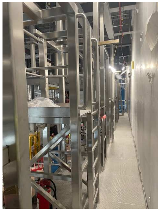
Astrazeneca Dublin. OMC installed stainless steel access platforms, Access stairs, Access ladders, lifting beams and galvanised access platforms.
