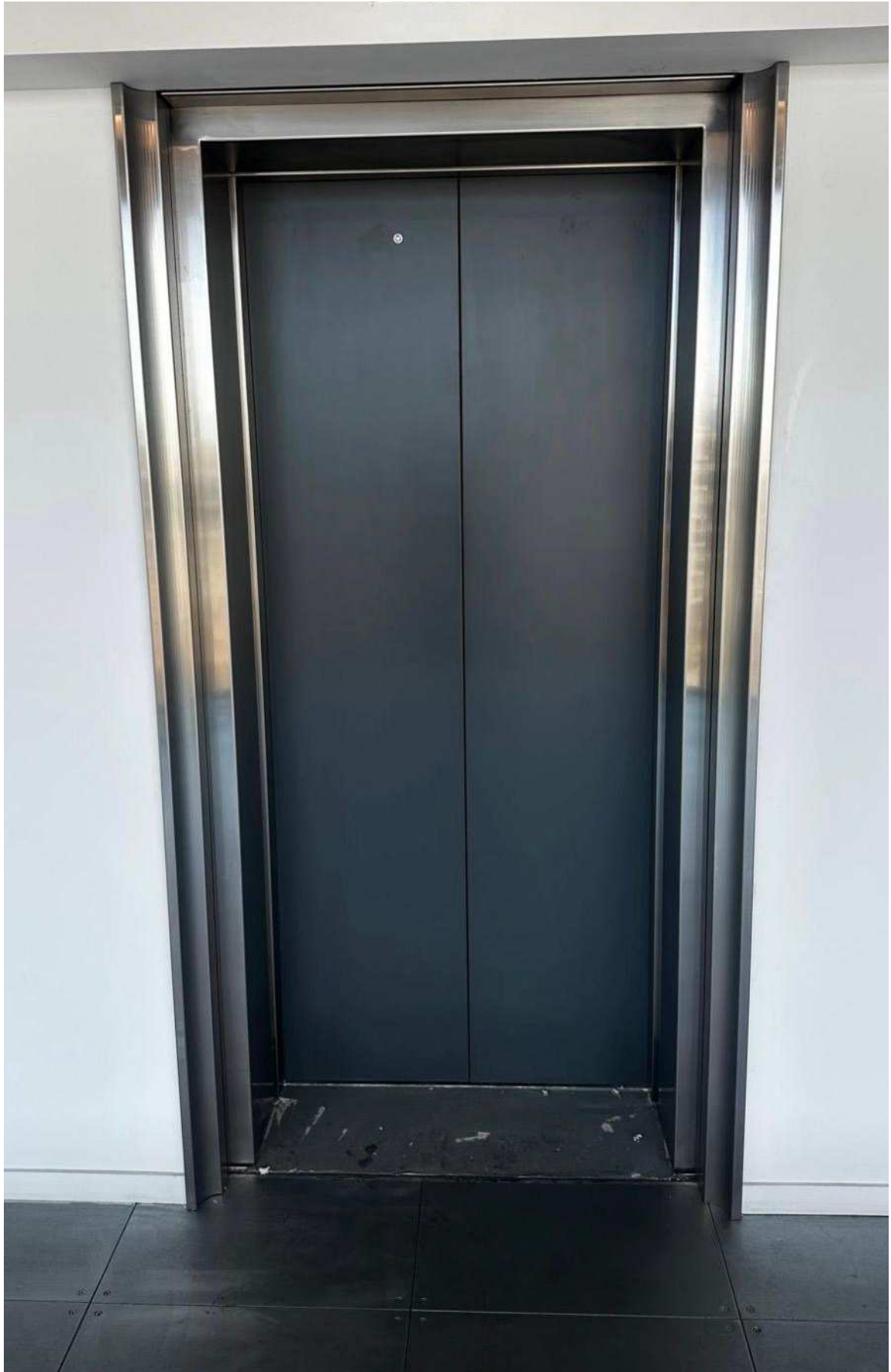
Polished stainless steel lift architraves with a radius quadrant on each side of the vertical architraves.
