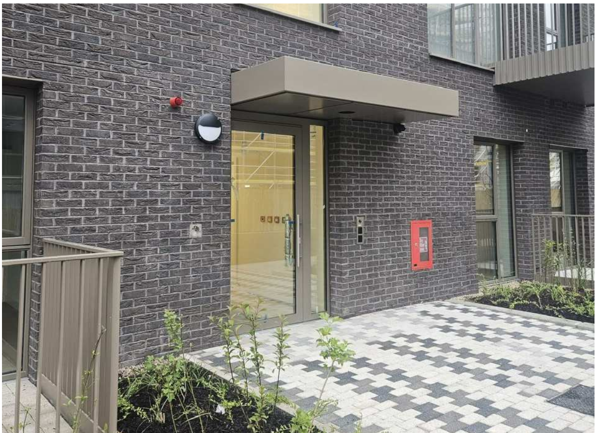
Galvanised and powdercoated railings, decorative privacy screens and entrance canopies installed in O 'Devaney Gardens Dublin.
