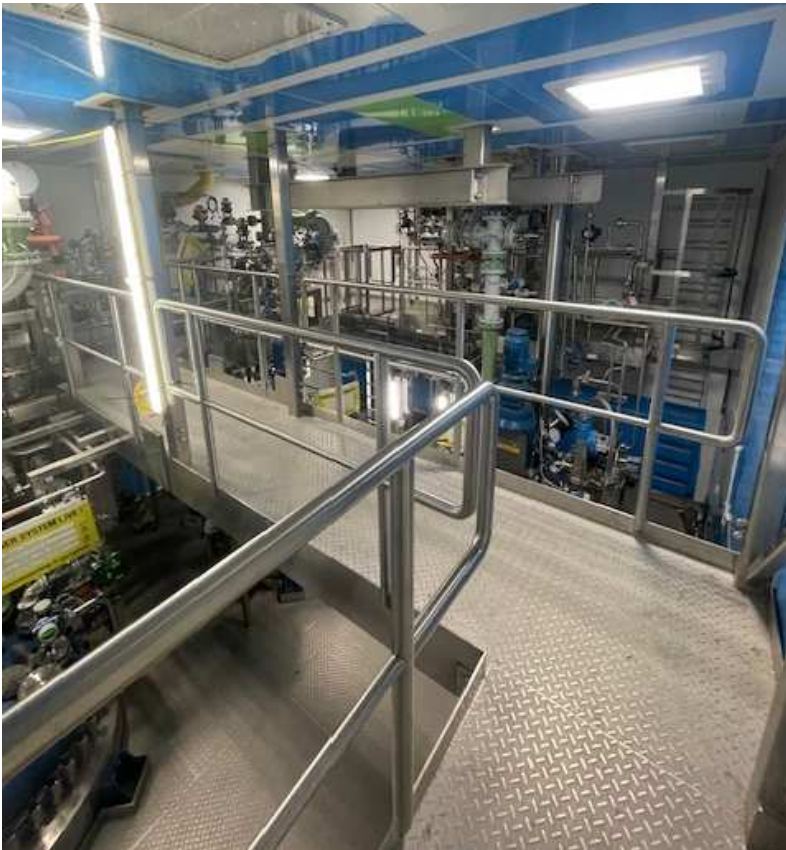
Astrazeneca Dublin. OMC installed stainless steel access platforms, Access stairs, Access ladders, lifting beams and galvanised access platforms.
