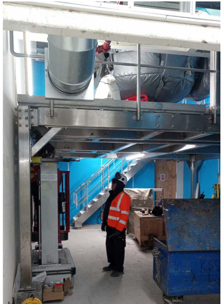
SK Biotek Dublin. OMC supplied & installed stainless steel access platforms, Access stairs, lifting beams and floor gullies.
