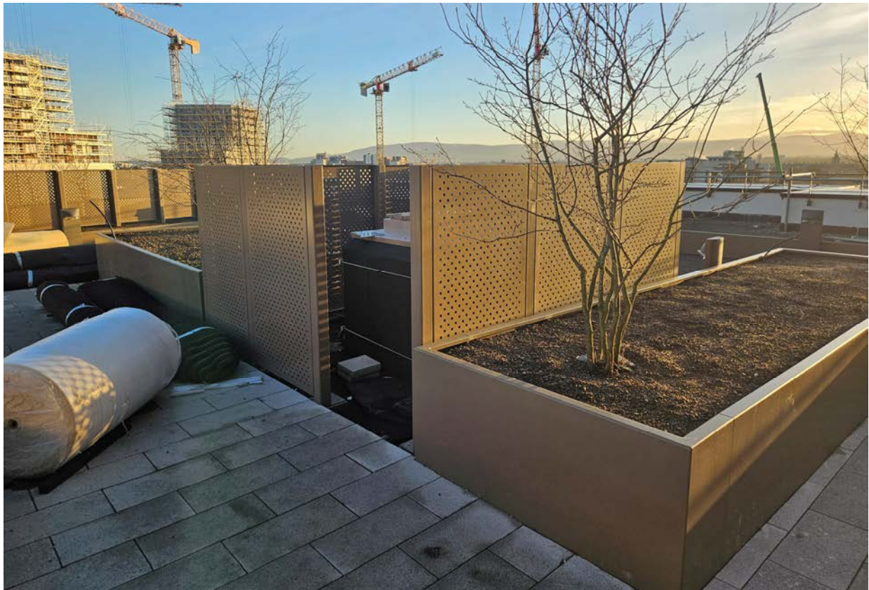
Ariel view of the apartments in O'Devaney showing various OMC steelwork elements and above photo showing planter boxes and perforated screens.
