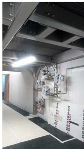
SK Biotek Dublin. OMC supplied & installed stainless steel access platforms, Access stairs, lifting beams and floor gullies.
