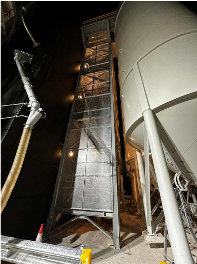
Galvanised perforated panels fitted to the external tower and outer side of the stairs.
